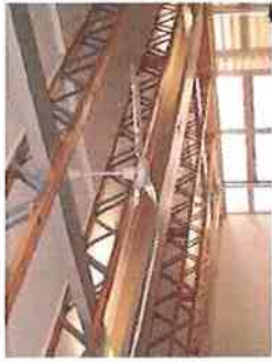
5 WOOD TRUSS STRUCTURE PHOTOGRAPH BY
